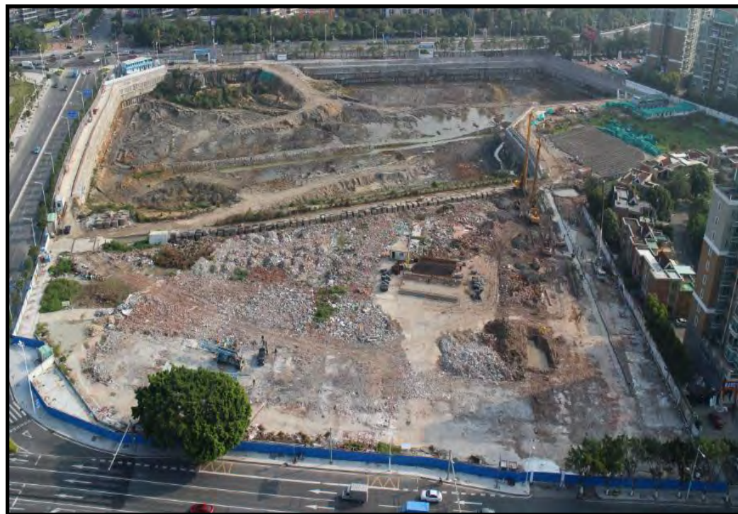
Site preparation works
