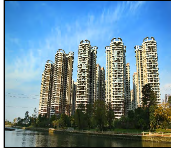
Millennium Waterfront Project, Chengdu, PRC
