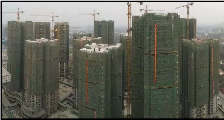
Plot A blocks under construction
