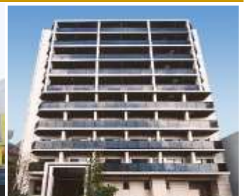
City Lux Yokohama (78 units)
