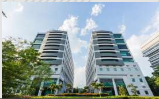
Citilink Warehouse (8 strata units)
