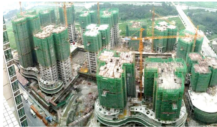
Aerial view of Plot A blocks under construction
