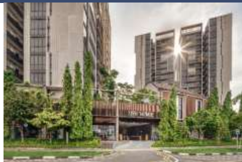
The Venue Shoppes & Carpark (11 strata units & one strata carpark with 82 lots)
