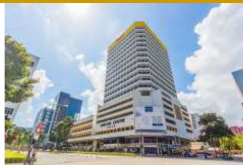
Fortune Centre (27 strata units)
