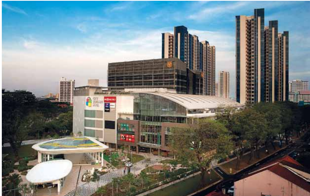
The first commercial development to be accorded a Building and Construction Authority (BCA) Green Mark Platinum Award, City Square Mall boasts of an extensive range of innovative green features.
