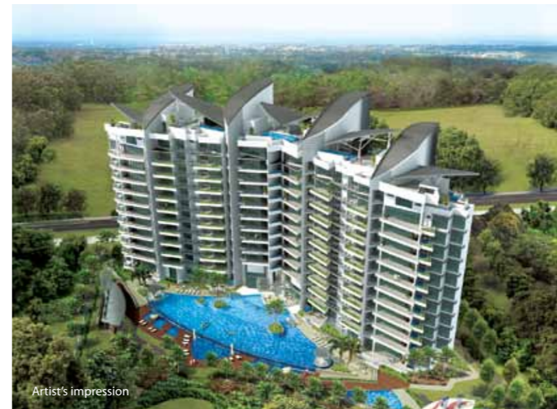
In line with CDL's CSR commitment to sustainable business practices, four CDL developments including Volari (above), were recently awarded the BCA Green Mark Platinum Award, Singapore's highest green rating for buildings.
