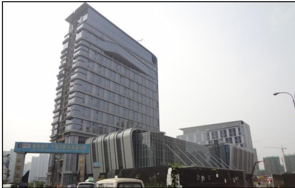
Crowne Plaza Chengdu Wenjiang and Holiday Inn Express Chengdu Wenjiang Hotspring hotels under construction
