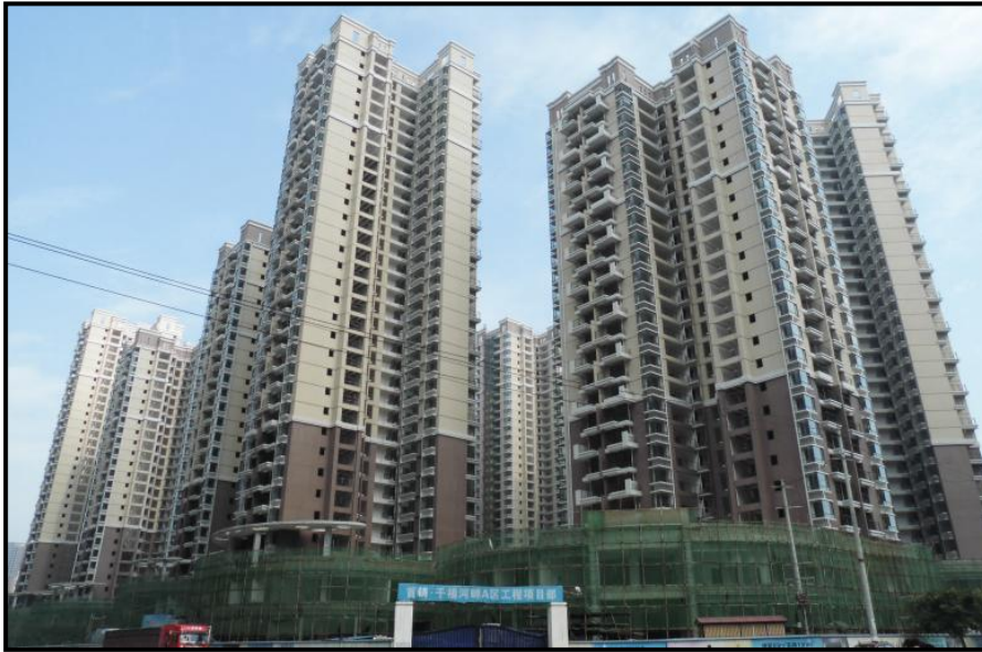
Plot A blocks under construction
