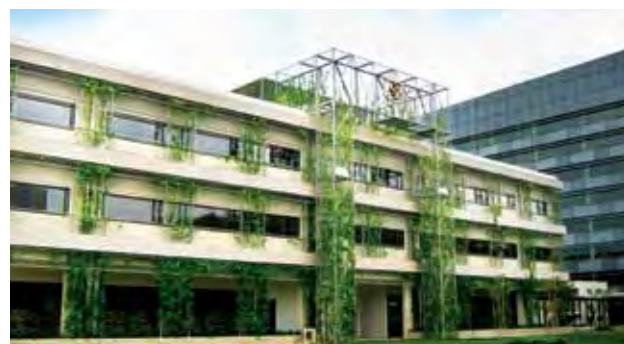
11 Tampines Concourse is the first building in Singapore constructed with extensive use of recycled materials for structural building components.
