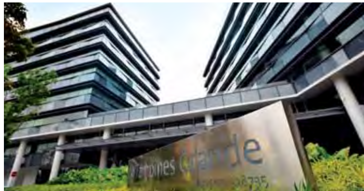
7 & 9 Tampines Grande is the first completed development in Singapore to achieve the LEED Gold certification under the Core & Shell Category.
