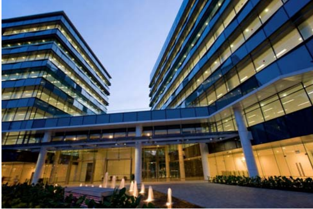
7 & 9 Tampines Grande 300,000 sq ft 8-storey blocks
