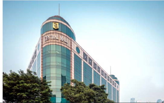
Central Mall (Office Tower)
