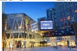
Nanping Starlight Place, Chongqing 重庆南坪星光时代广场
