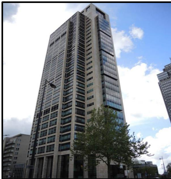
Mondriaan Tower, Amsterdam, the Netherlands
