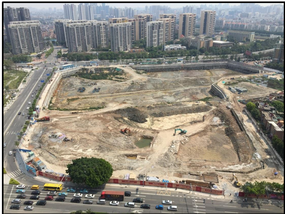
Site preparation works
