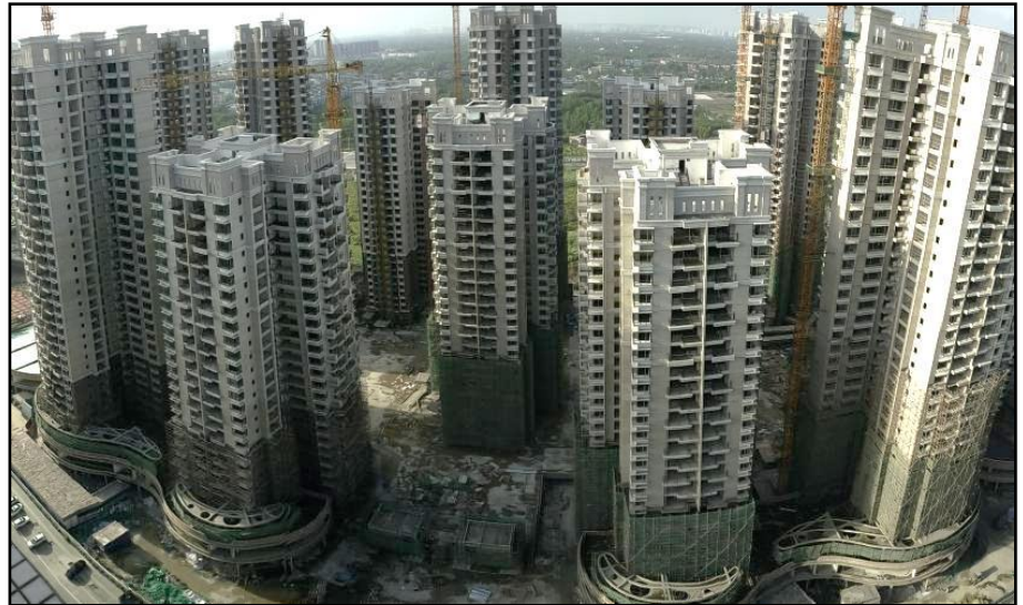
Plot A blocks under construction
