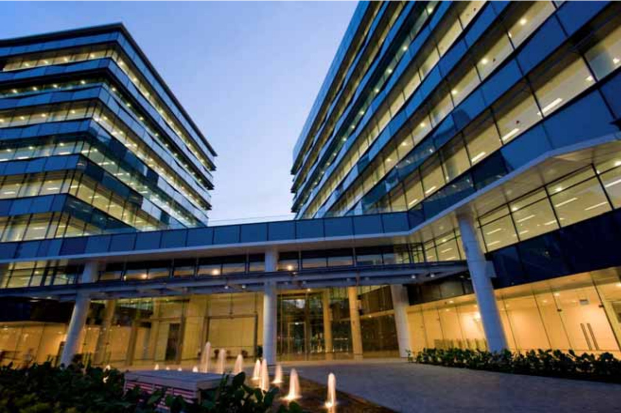
7 & 9 Tampines Grande 300,000 sq ft 8-storey blocks
