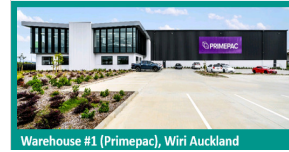
Warehouse #1 (Primepac), Wiri Auckland
