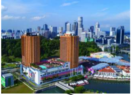
CanningHill Piers ^ (696 units)
