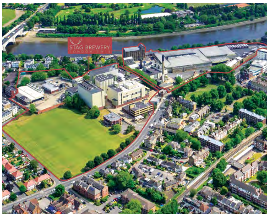
The expansive Stag Brewery land site is strategically located next to the River Thames and offers tremendous potential for redevelopment.
