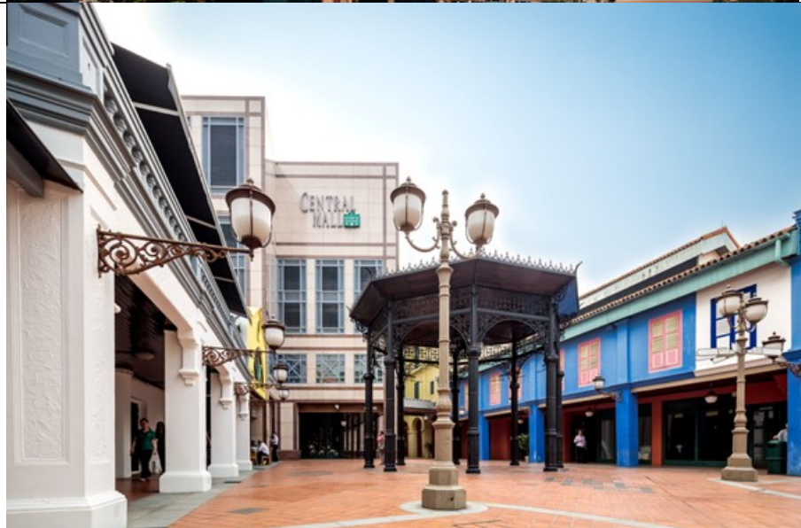
3 Central Mall (Conservation shophouses)
