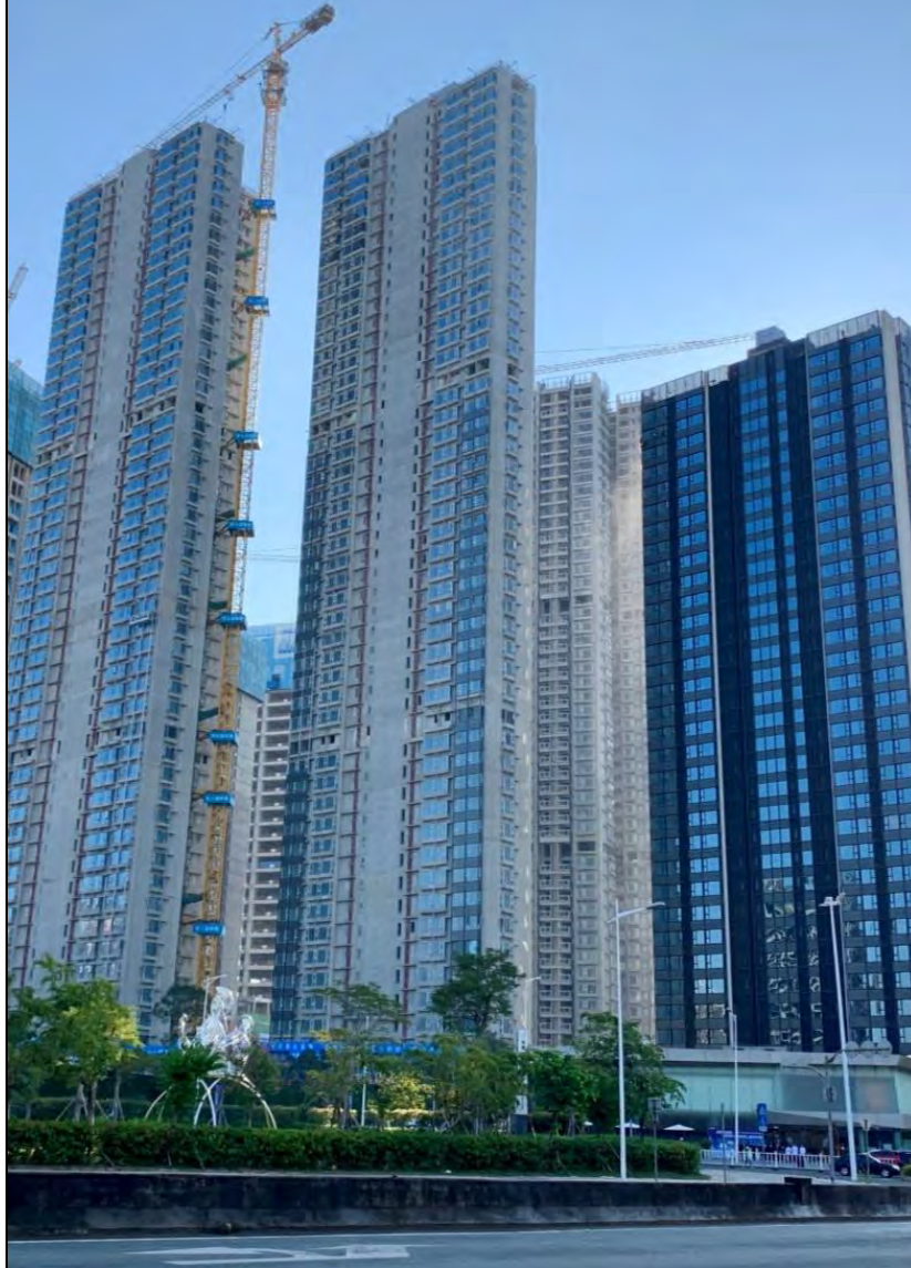
Star of East River Project, Dongguan Residential Blocks
