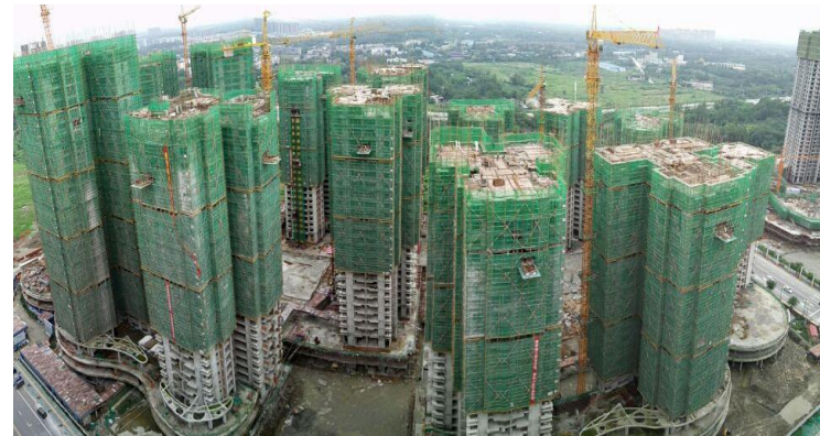
Aerial view of Plot A blocks under construction
