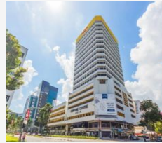
Fortune Centre (strata units)
