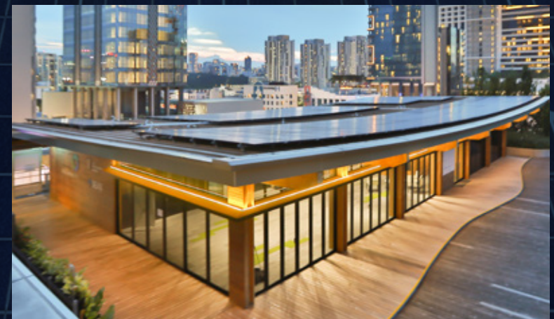
South Beach's microclimatic canopy covered with PV panels (top picture). Singapore Sustainability Academy (SSA) is a zero-energy and BCA Green Mark Platinum building opened in June 2017 (bottom picture).
