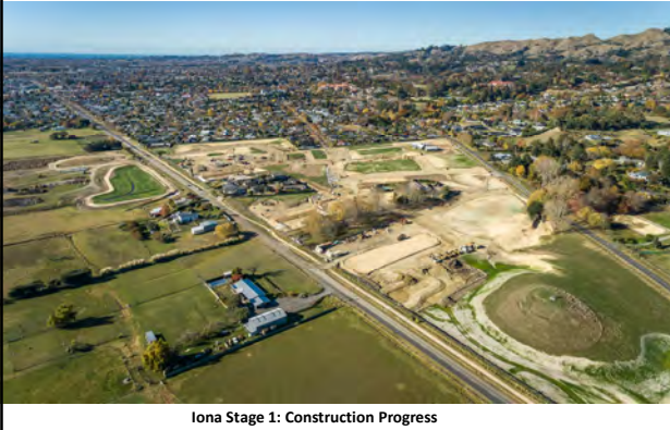
Iona Stage 1: Construction Progress
