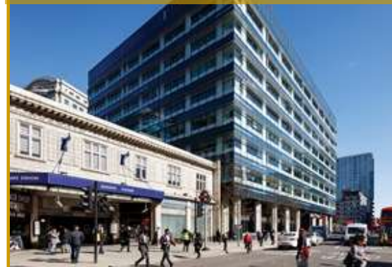
Asset Refurbishment @ Aldgate House
