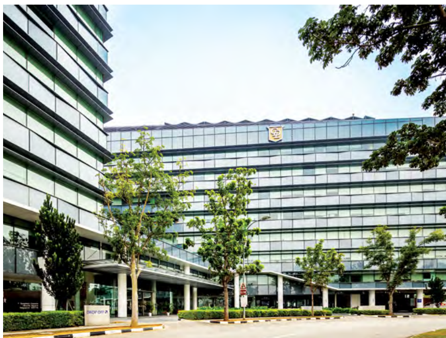
7 & 9 Tampines Grande is one of the three prime office assets in the portfolio of CDL's second PPS. The building has a net lettable area of around 288,000 sq ft.
