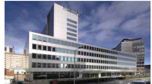
15 Lansdowne Road, Croydon
