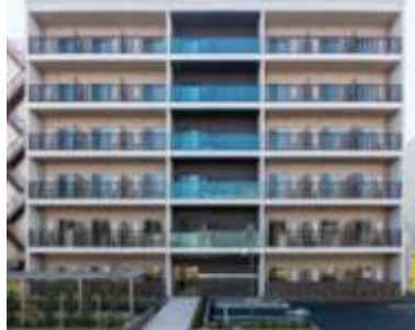
LOC's Yokohama Bayside (89 units)
